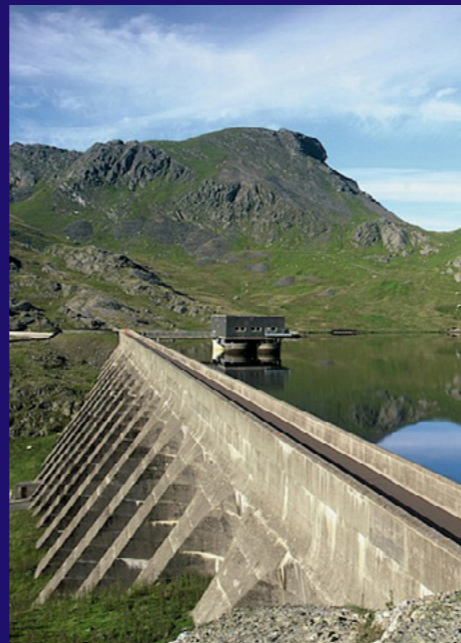
First Hydro Complex, North Wales
